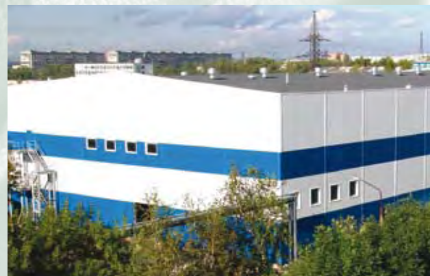
Johnson Matthey is the first western autocatalyst manufacturer to establish a plant in Russia. The facility shown is in Krasnoyarsk and will start operations in the first half of 2008.
