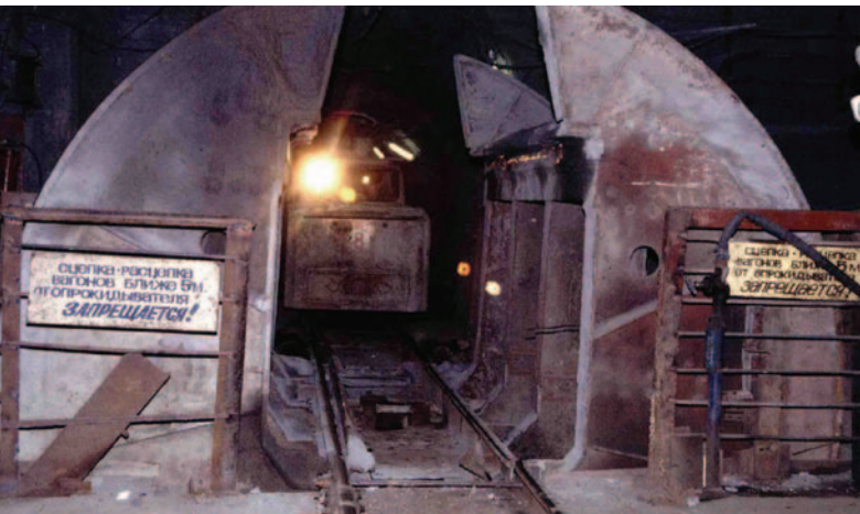
An ore transfer station at Norilsk's Oktyabrsky mine. Production of ore from the company's operations on the Taimyr Peninsula has stabilised at around 13 million tonnes per year.
