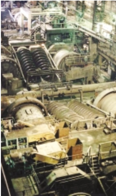
Part of the primary milling circuit at the Norilsk-Talnakh operations.
